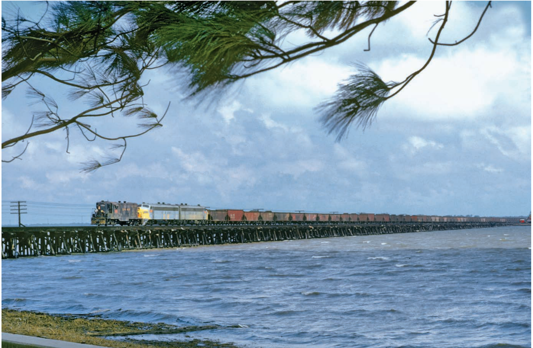
GP7 401 leads an FP7 and F7 on a long hopper car drag on the old timber version of the bridge at Bay St. Louis, Mississippi, in March 1964. The nearly two-mile bridge was replaced with a “hurricane-proof” structure made of prestressed high concrete in 1967, but subsequent storms have still inflicted some damage. L&N’s Gulf Coast line was always highly vulnerable to the giant storms. — I.W. King photo
